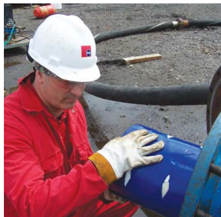
Foam pigging tool being loaded into pipeline
