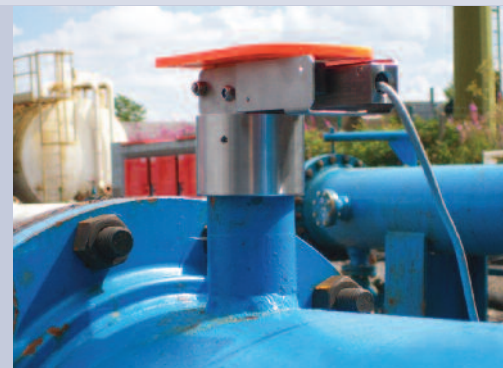
Pig signaller on pipeline
